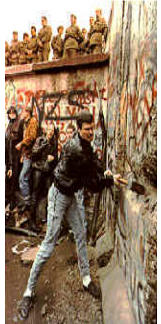
Tearing down the wall
